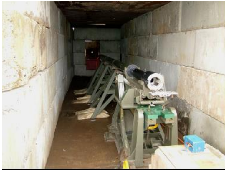
Figure 6: Gun protected in a bunker (courtesy of QinetiQ)
